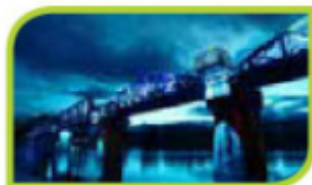
Kwai River Bridge
