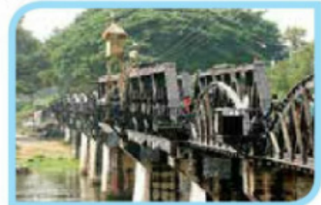
Kwai River Bridge
